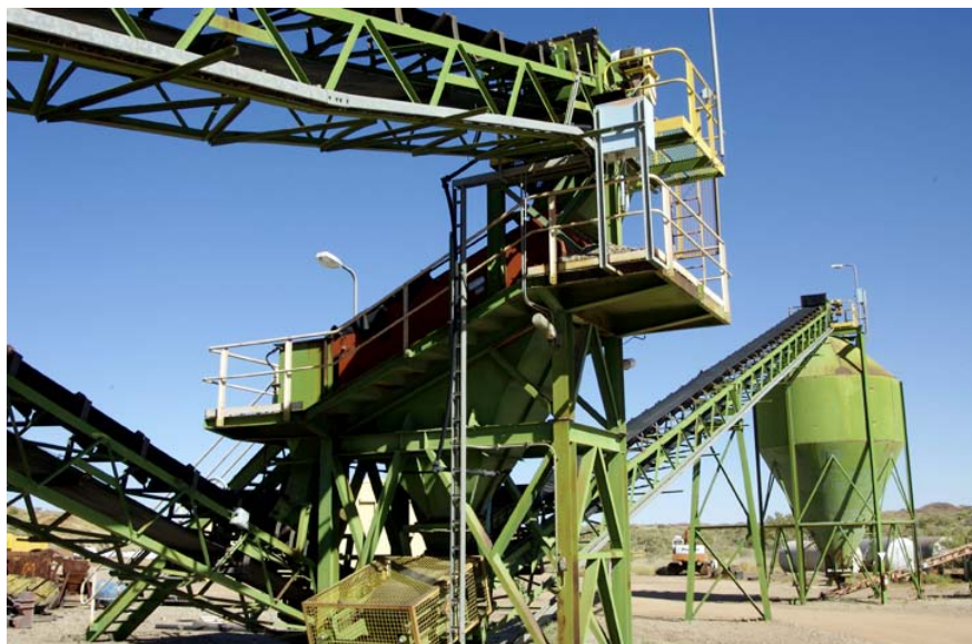
Fig. 3. Northwest's treatment plant
